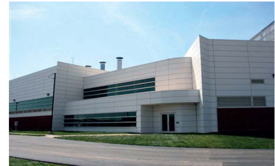
Central Utility Plant, Ft. Detrick, MD
